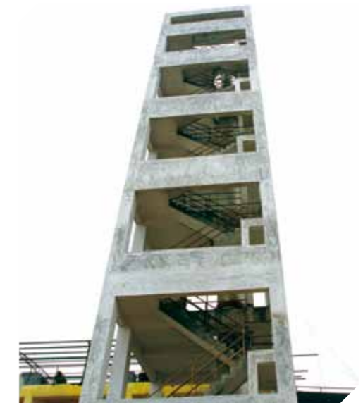
Tower stream ammonium device in service
