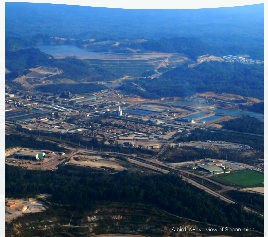
Almost all of Sepon's power requirements can now be met through renewable hydroelectricity
