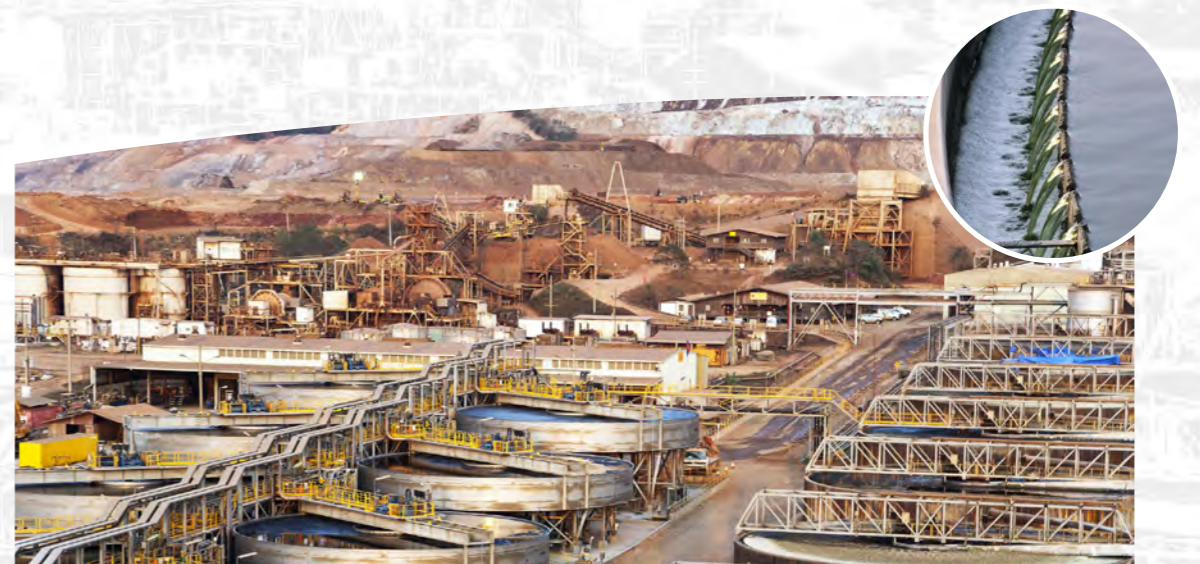
Wastewater treatment site at Sepon mine
