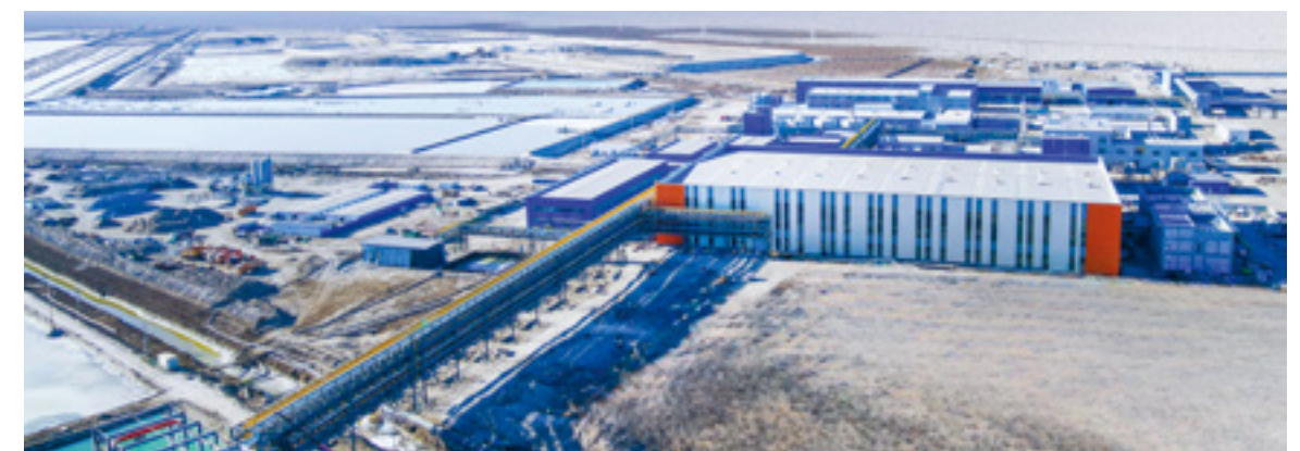
World's First 10,000-ton-level Industrial Demonstration Line for Lithium Extraction from Raw Salt-lake Brine
