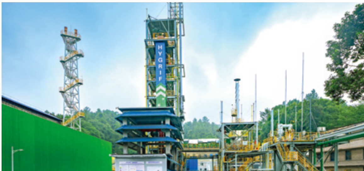
Hydrogen-based Shaft Furnace Project
