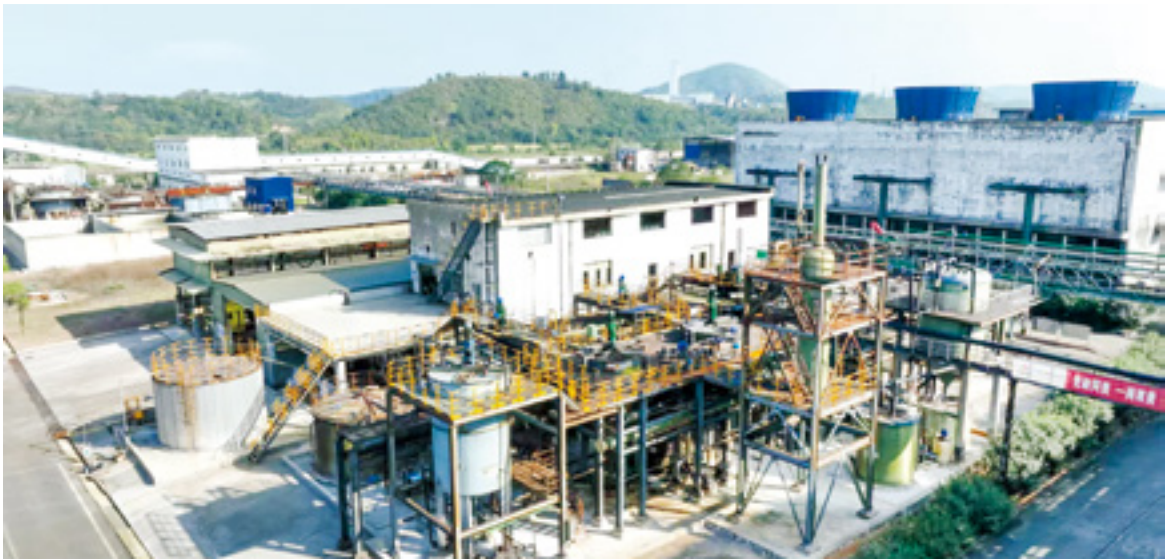
Acidic Wastewater Treatment Area of Minmetals Copper
