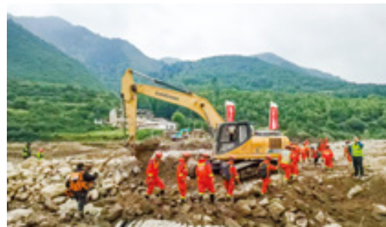
Emergency Construction of a Temporary Access Road to Duijiazhuang
