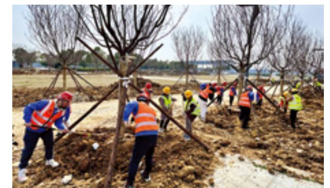
Greenery Planting Operations at China First Metallurgical Group’s Huangshi Daye Lake Project
