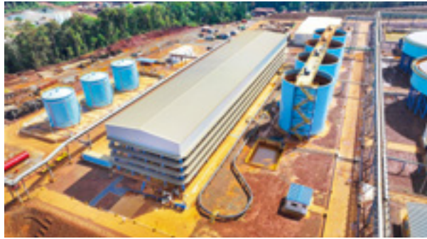
Key process technologies and equipment for long-distance slurry pipeline transportation - Large High-pressure Diaphragm Pump Station
