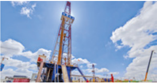
Development and Utilization of Medium-Deep Geothermal Energy by Shen Kan Engineering & Technology Corporation, MCC
