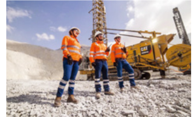
Workers at the Las Bambas Mine Open Pit
