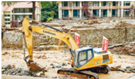
Dredging Rivers around S104 in Yuzhong County
