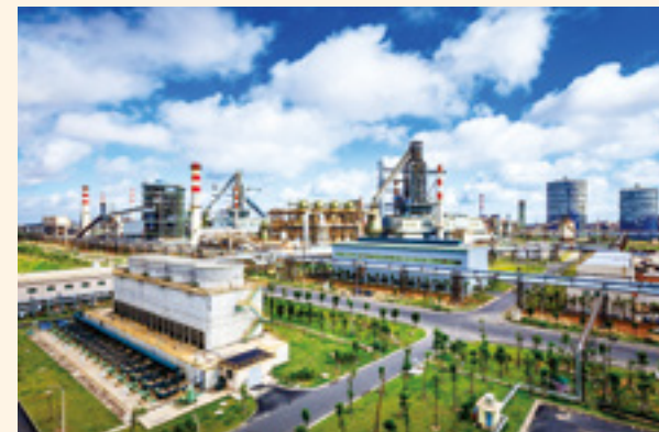
Baowu Zhanjiang Steel Project
